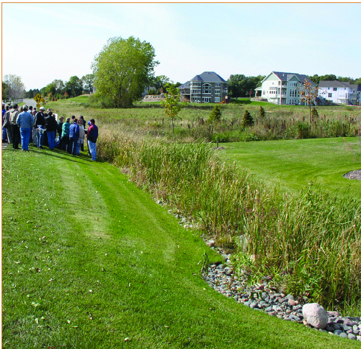
A road ditch can serve as a bioswale. The rock trench and wetland vegetation are notable features, along with the natural drainageway in the background that serves as a bioswale for residential runoff.
