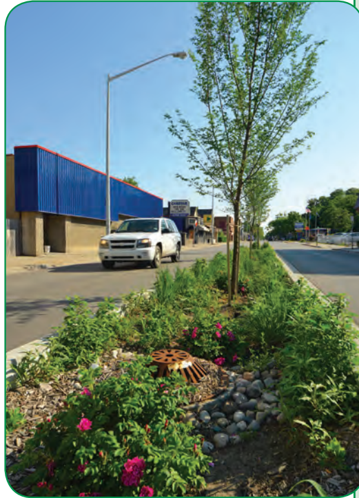
Plainfield Avenue, Grand Rapids, Michigan linear bioretention.
