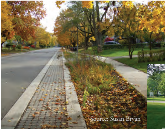
(Left) Easy Street after and (below) before construction.
