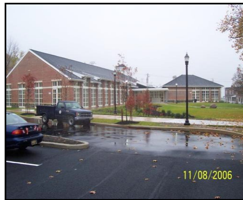
Porous asphalt parking lot in Wilm., DE
