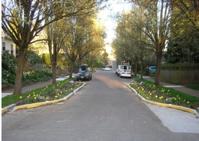
Residential application of a vegetated curb extension in Portland, Oregon (Source: www.artfulstormwater.net )
