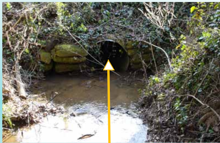
Undersized pipe culvert
