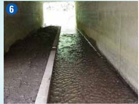
photo: Brad Ehrman, GDOT
