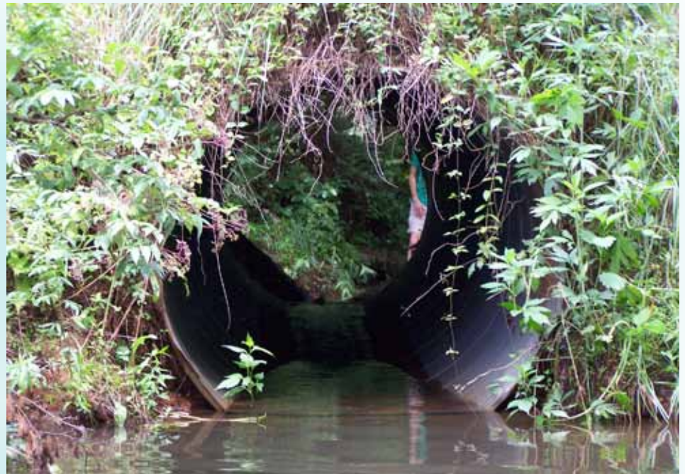
Cochran Creek tributary, Dawson County. Impassable to fish because water is shallow, fast, and downstream end is perched.
