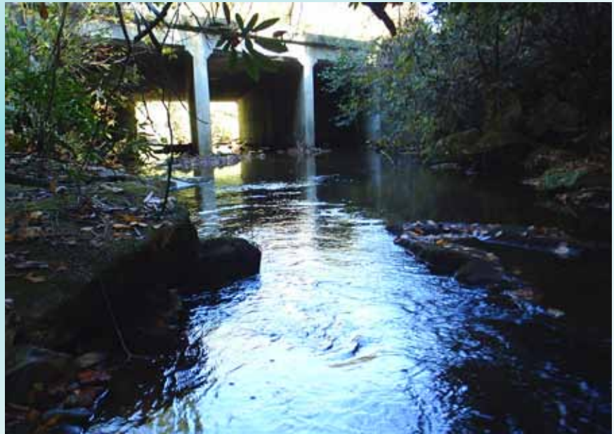
Fish passable box culvert over Fightingtown Creek in Fannin County. Photo courtesy of Brad Ehrman GDOT.
