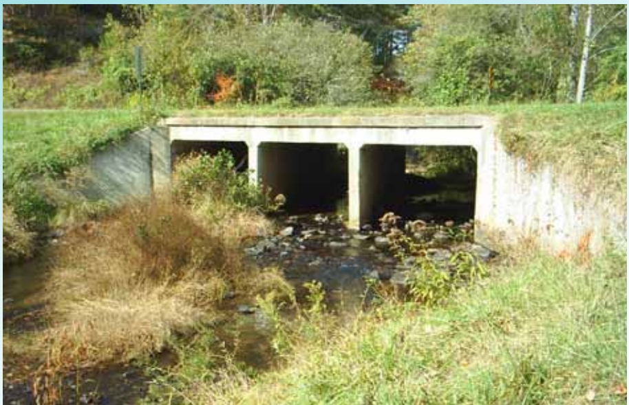
Top and bottom photos are fish passable culverts over Conasauga Creek, Gilmer County, GA. Photo courtesy of Brad Ehrman GDOT.
