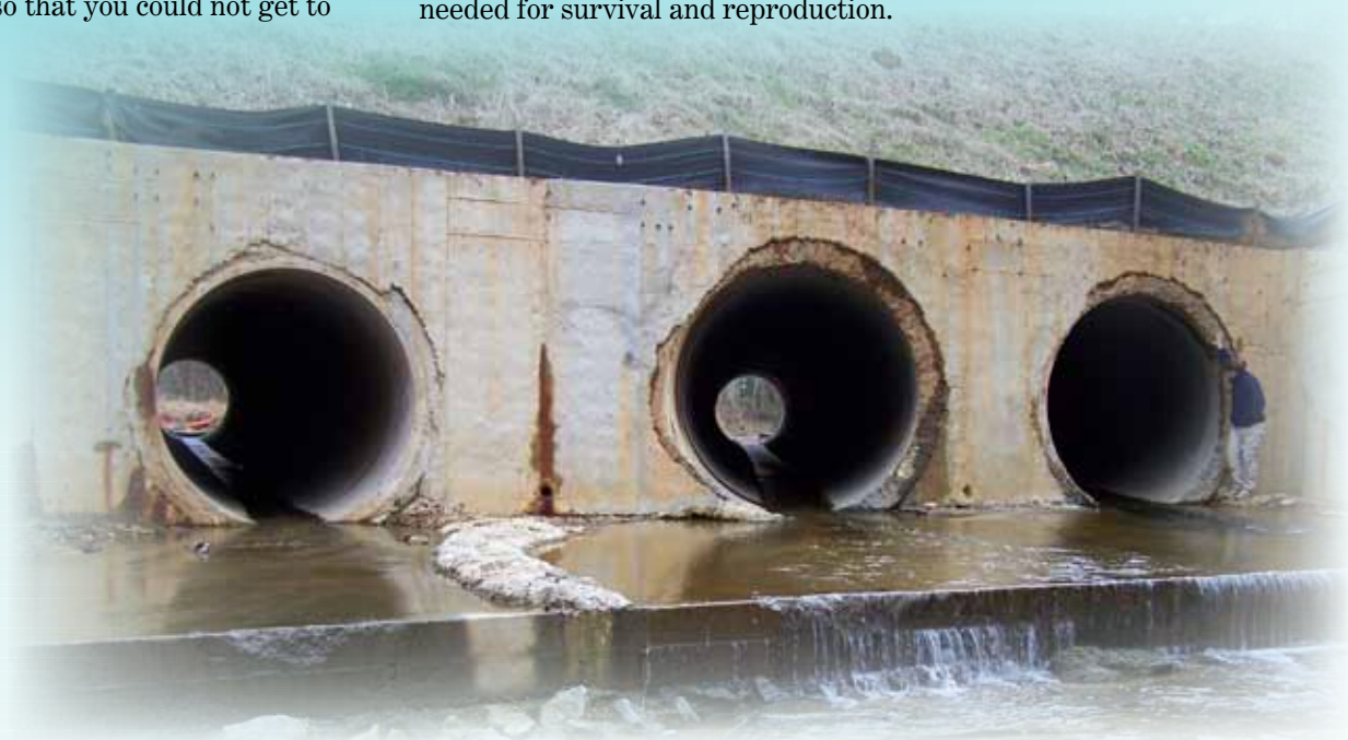
Flat Creek in Dawson County. Culvert is impassable to fish because it is perched and because water depths are too shallow.
