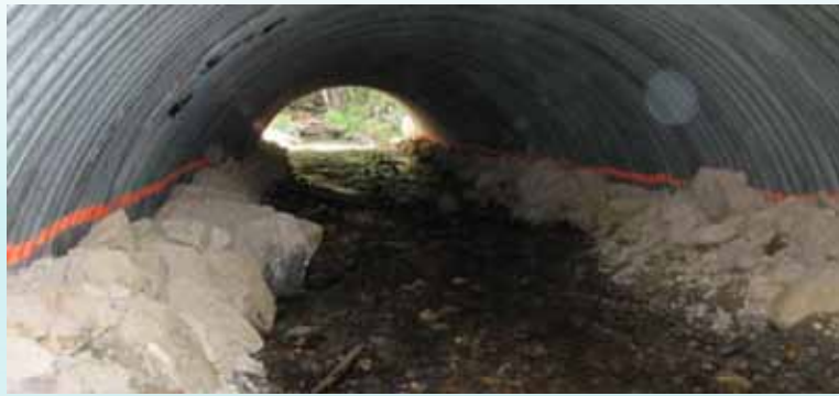
Low flow channel in an open bottom structure. Photo courtesy of USDA 2008a.
