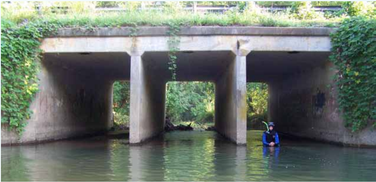
A culvert on Rock Creek, Murray County. Culvert is impassable to fish due to shallow water inside culvert and because it is perched on the downstream side.
