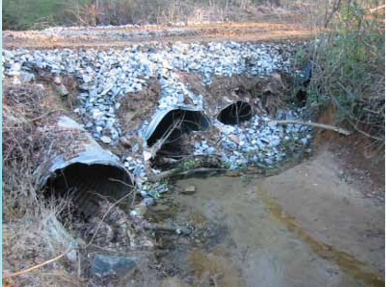
South River tributary, Clayton County
