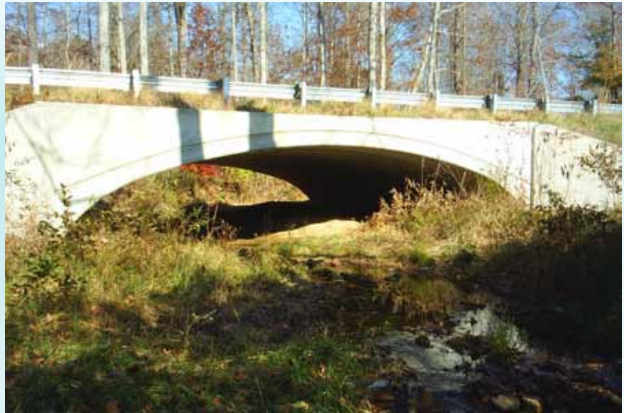
Fish passable arch-span culvert over a Shoal Creek tributary in Cherokee County. Photo courtesy of Brad Ehrman GDOT.
