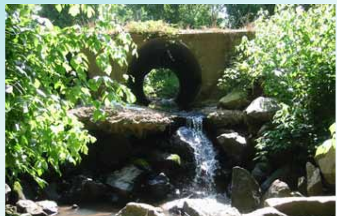
Tributary to Little Sugar Creek, Morgan County. Impassable because outfall is perched above creek. A longitudinal stream profile would show a significant difference in upstream and downstream bed elevations.
