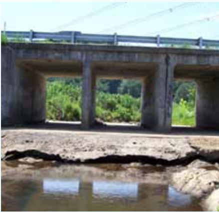
Raccoon Creek in Paulding County, Probably impassable because water flows under the concrete foundation, not through the culvert.
