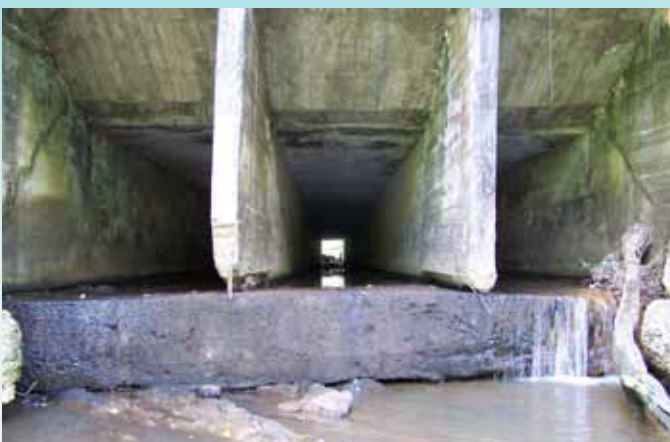
Raccoon Creek in Paulding County. Impassable because of shallow water depth and perched above creek.
