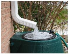
Rain Barrel Inlet Filter
