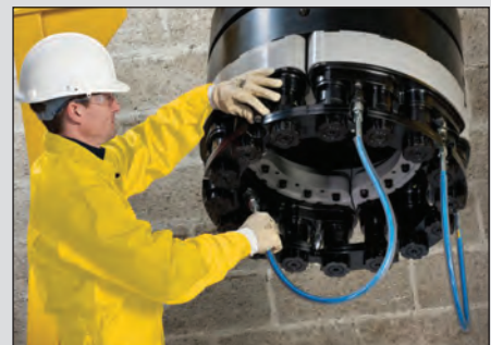
▲ Multi-Stud Tensioning application.
