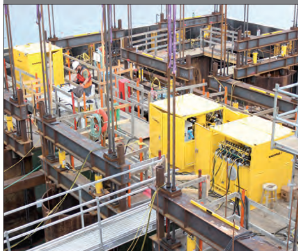
▲ Custom hydraulic pump for a bridge deck launching system.
