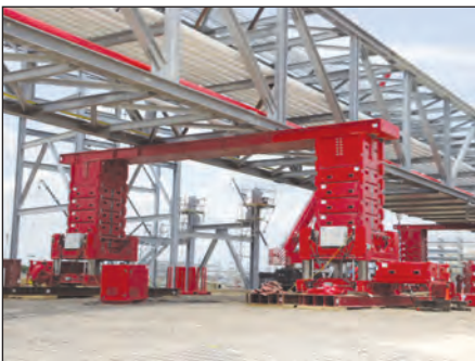
▼ Lifting an oil and gas pipe module
