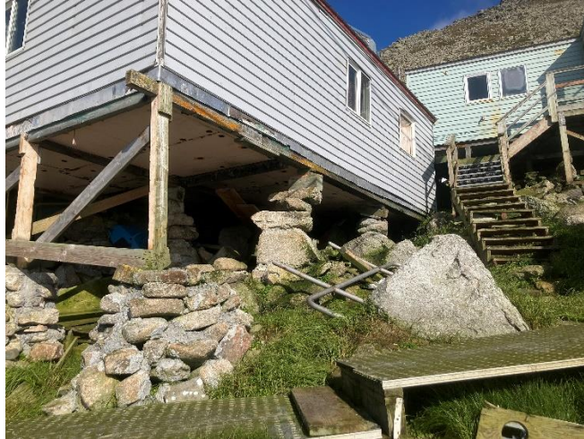
Figure 2 Example of Foundations Observed
