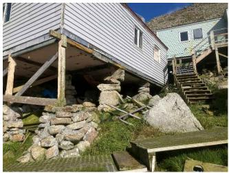
Figure 2 Example of Foundations Observed
