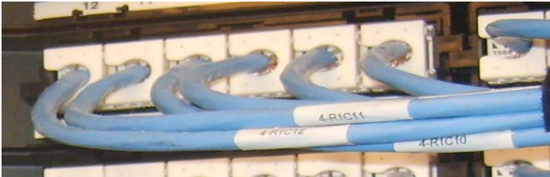
Patch Panel Rear View (Close Up)
