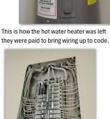
They were paid to install a new electrical panel box but this is the same one we've always had. There are issues, one breaker trips each time it's flipped. We have dead plugs and switches throughout the house that were not like that prior. Their painter painted over the wires & breakers while
