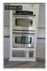
The ovens have no power, their wires are hooked up to the sources and the source has power but the ovens have no power. Electrician will have to pull them and address issue.
