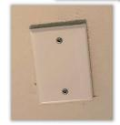
There are plugs and light fixtures that are no longer usable because they removed the light fixtures and outlets and put blank plate covers in their places.
