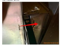
Monitor: Some evidence of prior condensate leakage was noted on the unit. This condition requires close monitoring.
