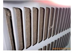
Upgrade: Recommend vegetation be cut back to provide three feet of clearance from the unit.
