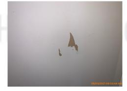
Monitor: Water staining was noted in the kitchen. The stain tested dry with a moisture meter at the time of inspection.
