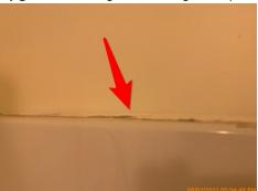
**Upgrade:** Cracked, deteriorated and/or missing shower stall grout and caulk should be replaced.
