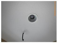
**Monitor:** Recessed light fixtures (sometimes referred to as pot lights) that are installed in insulated ceilings can represent a fire hazard if they are not suitably rated for this application. Unfortunately, it is difficult to verify that the installation has been made safely, during a home inspection. It is recommended that a licensed electrician be engaged to verify the safety of the system.
