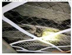
**Upgrade:** The air filter for the supply air has been inserted backwards. The air flow arrow should point towards the furnace unit.
