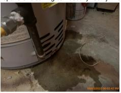
Monitor: The water heater shows evidence of prior leakage. This should be carefully monitored.
