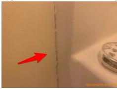
**Upgrade:** Caulking is needed around the shower controls. This will aid in preventing water intrusion into the walls.
