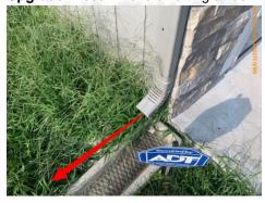
**Upgrade:** The downspout rear right corner has been damaged. Replacement is recommended.
