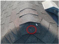
**Monitor:** The roofing is considered to be in fair condition. This roofing is wearing at uneven rates. The sides of the roof that are most exposed to the sun s light are wearing more quickly than the more shaded areas. Repair or replacement of deteriorated roofing may be needed in some areas, prior to the entire roof covering requiring replacement.
