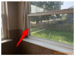
**Upgrade:** Water stains were observed on some of the window sills. Sealing or painting windows to protect against the elements is recommended.
