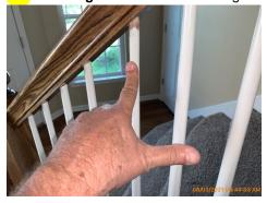
WRN: Warning: The loose handrail should be better secured.
