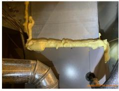
**Upgrade**: The skirt over the flashing for the exhaust flue should be caulked to prevent further water streaking down the outer skin of the flue in the attic.
