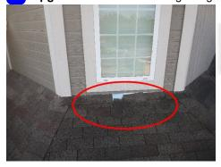
**Upgrade:** Nail heads are exposed. Recommend sealing fasteners.
