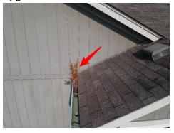
**Upgrade:** The gutters are leaking at some of the joints. Recommend the joints be repaired, patched and sealed.
