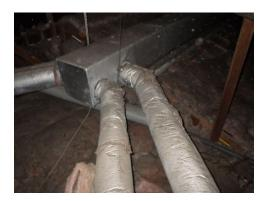
Observed dirt/debris etc inside return air chase. We recommend remove/clean debris from return. To minimize air/dust infiltration, seal drywall joints as required according to today's standards.
