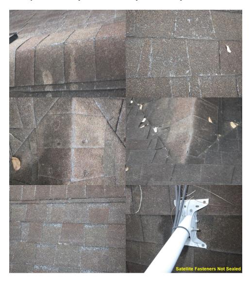
Damaged (broken, torn etc.) shingles were observed caused by contact with trees. We recommend further inspection by a specialist contractor and repair or replace as necessary to prevent water penetration.
