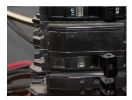
The circuitry in the electric service panel was not properly labeled. We recommend that every circuit be identified and labeled, allowing individuals unfamiliar with the system to recognize the locations of each circuit.
