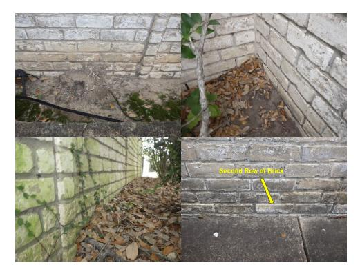
Soil grading had depressions or inadequate / negative slope in some areas and did not appear to properly direct runoff water away from foundation as required according to today's standards (6" drop in 10' Ref: IRC 401.3). This may promote water penetration, adversely affect the foundation and cause differential settlement. We recommend repair as necessary.
