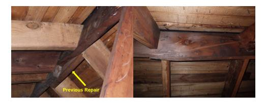
Some sag or unevenness in roof decking observed at front / right side of house. Probable cause from improper/inadequate framing in attic. (This is common where wood shingle roof with skip sheathing has been covered with solid decking and composition shingles.) We recommend installation of stronger purlins with bracing down to load bearing walls to arrest further movement/sagging of roof.
