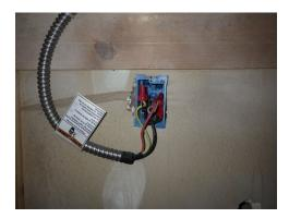
Exposed and improper wiring was observed in garage. This is a potential shock and fire hazard. We recommend further inspection by a licensed electrician and repair or replace as necessary.
