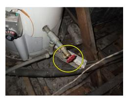
The water heater Temperature & Pressure relief valve drain line was not an approved material. Flex connectors reduce pipe diameter and can improperly restrict flow. We recommend replace drain line with material approved according to today's standards.
