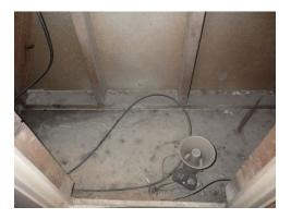
Observed 120 volt electrical wiring located in return air chase. According to today's standards (code) 120 volt wiring should not be located in, or pass through chases. In the event of an electrical fault / fire, this could promote spread of fire into attic. This may have been allowed at the time of construction, but for enhanced safety, we recommend alteration if possible.
