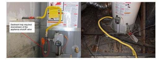
The drain line for water heater drain pan had improper connection. This may promote
