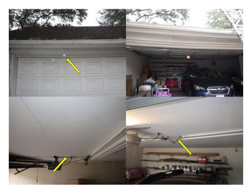
Frieze board or eave separation was observed at one or more corners of house. This is frequently an indicator of movement in the structure. We recommend secure / seal gaps to prevent water penetration.
