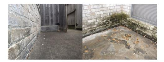
There are one or more trip hazards throughout the walkways / patio / driveway. A trip hazard is defined as an irregularity in a walking surface exceeding one inch in height. We recommend they be patched or repaired to provide an even walking surface.
