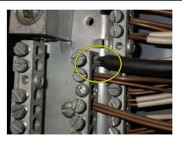
Multiple conductor cables were loose where entering the electric service panel. We recommend the cable be secured by installing an approved connector as required according to today's standards.
