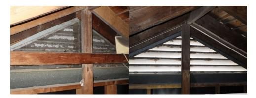
Attic insulation was minimal by today's standards. The insulation has been compressed and/or been disturbed insome areas and no longer provides the same R-value as when it was installed. We recommend reposition or add more insulation to increase energy efficiency.
