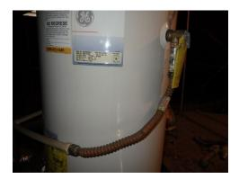
The water heater gas piping did not include a drip leg (sediment trap) extension to collect contaminants (sediment, debris etc) as required according to today's standards. For enhanced safety and proper operation, we recommend alteration as required according to todays standards (Ref: IRC G2419.4) and manufacturer's recommendations.
