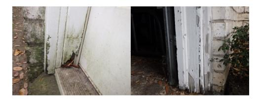
Observed what appeared to be sagging of header (support beam) over garage door and sag in garage ceiling. This can be caused by movement in the structure and/or deteriorated or improper framing. We recommend further inspection by a specialist contractor and repair or replace as necessary.
