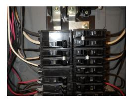
There was no anti-oxidant compound (grease) visible on an aluminum connection as required by TREC and many manufacturers. Antioxidant is applied to aluminum connections according to manufacturer's recommendations to prevent oxidation, electrical resistance and heat. We recommend apply antioxidant as necessary.
