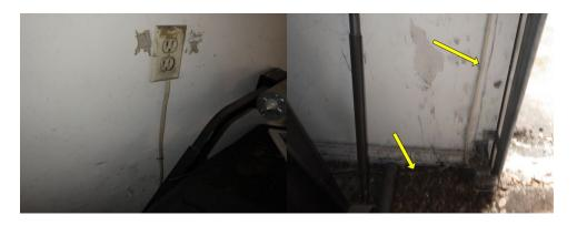
Observed extension cord wiring in attic used improperly as permanent wiring in one or more areas. This is a possible fire hazard. We recommend further inspection by a licensed electrician and repair or replace as necessary.
