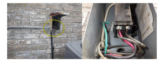
We found overfusing in the main electrical service panel, meaning the conductor was inadequate size to safely carry current allowed by the circuit breaker. This is a potential fire hazard. We recommend the circuit be equipped with a properly rated conductors and/or circuit breaker.
