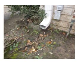
The gutters were damaged in one or more areas, had accumulated debris preventing proper drainage. We recommend all debris be cleared.
