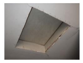
Ceiling cracks and wrinkled drywall taper were observed in some areas. (Photos are examples only and do not represent all instances of condition.) This may be an indication of movement in the structure. We recommend repair for cosmetic reasons and monitor for changes.
