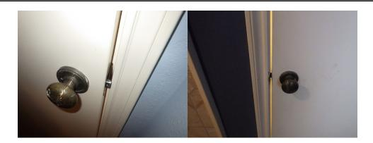
The door from house to garage was not square, had a gap at top, meaning it was not a fire resistant assembly as required to protect an opening between garage and dwelling (Ref: IRC R302.5.1). A solid core wood or honeycomb steel door 1 3/8" thick minimum or UL listed 20 minute fire rated door with self closer is required. We recommend install fire resistant door with self closer as required according to today's standards.
