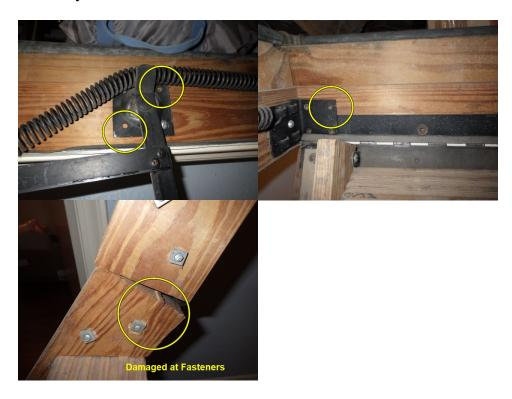
The folding attic stairs did not close properly. We recommend repair to seal gaps and prevent loss of conditioned air to attic and/or sucking attic air into house. As an upgrade, we recommend weather stripping and insulating stairway if not done already.
