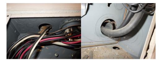
The hot & cold metallic water piping did not appear to be properly bonded to gas piping and the house grounded service at main panel as required according to today's standards. This may not have been required at time of construction, but to minimize shock hazard in case of ground fault, we recommend install bonding connections. (Ref: IRC E3509.7)
