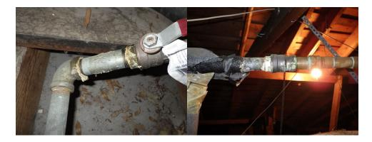
Observed water heater vent pipe(s) not properly secured (strapped) to roof rafters in attic. Strapping gas appliance vents is required to resist wind storm damage / disconnection of vent when wind pushes on vent and cap above roof line. We recommend repair as necessary.
