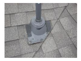
Caulking was observed to be missing or deficient on the storm collar above roof line for water heater and furnace vent. The storm collar protects the joint between a gas appliance vent pipe and roof flashing. We recommend caulking to prevent water penetration into attic.
