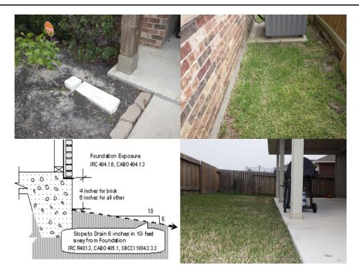
The drainage swale was not continuously sloped to street as required according to today's standards, may cause water ponding at side(s) of house. We recommend repair as necessary to promote proper drainage away from foundation and extend service life of fence.
