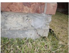
Observed uneven surface at foundation edge / aggregate visible. This is primarily a cosmetic condition, no repair recommended.
