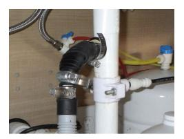
The dishwasher drain line lacked a visible backflow preventer (air-gap or high loop) as required by present standards and necessary to prevent mixture of supply and waste water from disposal. We recommend a high loop or an approved backflow preventer be installed.
