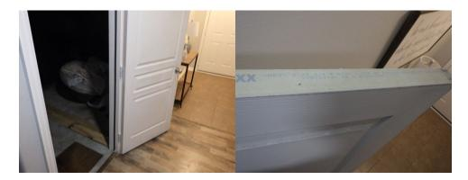
The front door was not square in jamb, improperly rubs frame. We recommend repair / adjustment to restore door(s) to a serviceable condition. This may be an indication of foundation movement or improper installation.
