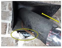
An unused / abandoned exhaust fan backdraft damper was visible over master bedroom. We recommend cover and seal to prevent water penetration.
