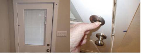
(work in progress) Temporary hardware was present in front door with no deadbolt. We recommend complete installation.
