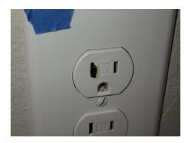
GFCI protection was not observed at 120 volt receptacles in laundry room, considered a wet/hazardous location according to today's standards. This may not have been required at the time of construction, but to minimize shock hazard, we recommend install GFCI protection.
