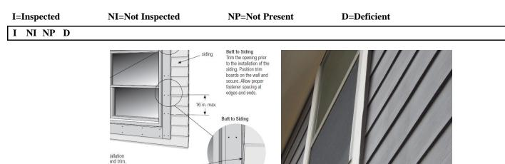
Observed caulking missing or deficient around wall penetrations in one or more areas. We recommend all wall gaps for trim over front entry / windows / plumbing / electrical etc, be caulked to prevent water penetration.
