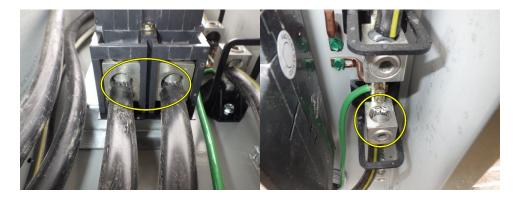
The system neutral and grounding conductors appeared to be improperly bonded together in garage subpanel. This can create two paths to ground and a create a shock and/or fire hazard in case of ground fault. We recommend further inspection by a licensed electrician and repair or replace as necessary (Ref: IRC E3607.2). We recommend further inspection by a licensed electrician and repair as necessary.
