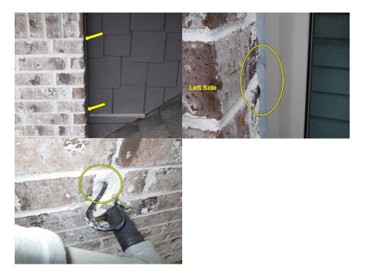
Observed gap in wall below flashing where air conditioner refrigerant / electric supply lines pass through exterior wall. We recommend install mortar and foam sealant to prevent water penetration and rodent entry.
