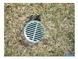
Soil grading had a depression or inadequate slope at rear, did not appear to properly direct runoff water away from foundation as required according to today's standards (6" drop in 10' Ref: IRC 401.3). This may adversely affect the foundation and cause differential settlement. We recommend repair as necessary.
