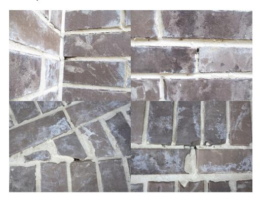
Caulking was observed to be missing from expansion joint(s) and / or inside corners of brick veneer in some areas. Ensure any mortar present in expansion joint is first removed before sealing with backer rod to allow movement.
