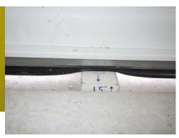
The garage door's infrared reversing beams were installed too high (more than 6") above the floor which decreases the devices effectiveness in preventing entrapment or injury. We recommend the beams be lowered to between four and six inches above the floor.
