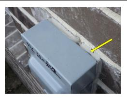
Observed gap in wall below flashing where air conditioner refrigerant / electric supply lines pass through exterior wall. We recommend install foam sealant and/or metal mesh to prevent rodent entry.
