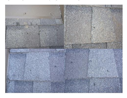
Observed shingles improperly installed, lifted/loose at lower edges in some areas. Loose shingles are prone to water penetration and more likely to be damaged in a windstorm. We recommend repair or replace as required according to manufacturer's requirements to prevent damage and water penetration. (The following example is from GAF installation instructions.)
