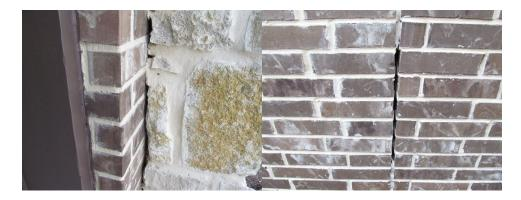
Observed caulking was missing or deficient around wall penetrations in some areas. We recommend all wall gaps for joints between cladding materials / vents / plumbing / electrical etc, be caulked to prevent water penetration.
