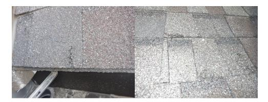
Observed multiple nail holes in shingles. These are likely from use of toe boards (lumber improperly nailed to roof surface to create walkway during construction). We recommend repair or replace as necessary to prevent water penetration.
