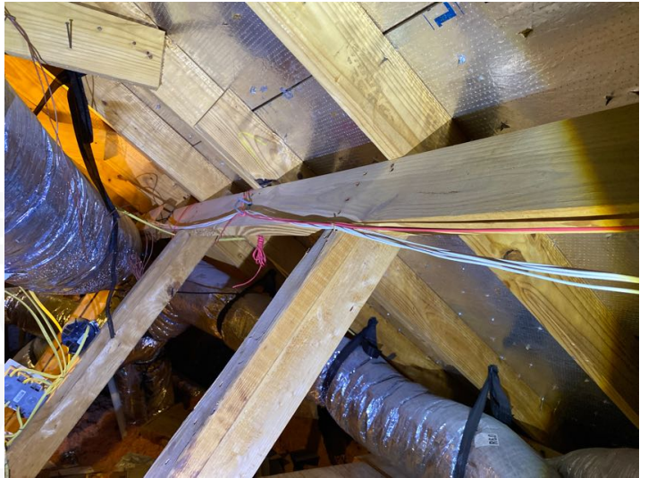
Roof Structures and Attic space
