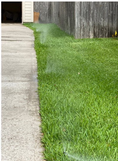
OPTIONAL SYSTEMS Landscape Irrigation (Sprinkler) Systems
