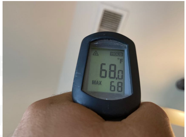
Delta T test at the register vent(upstairs)
