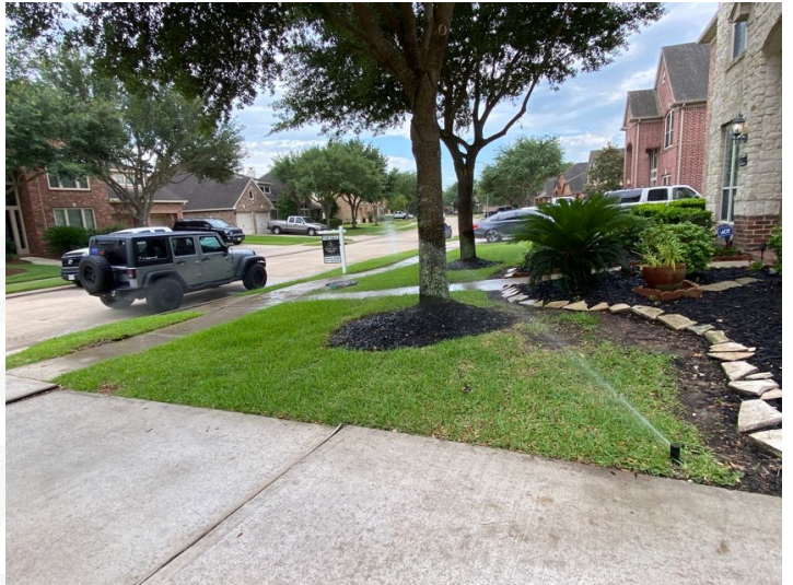
OPTIONAL SYSTEMS Landscape Irrigation (Sprinkler) Systems
