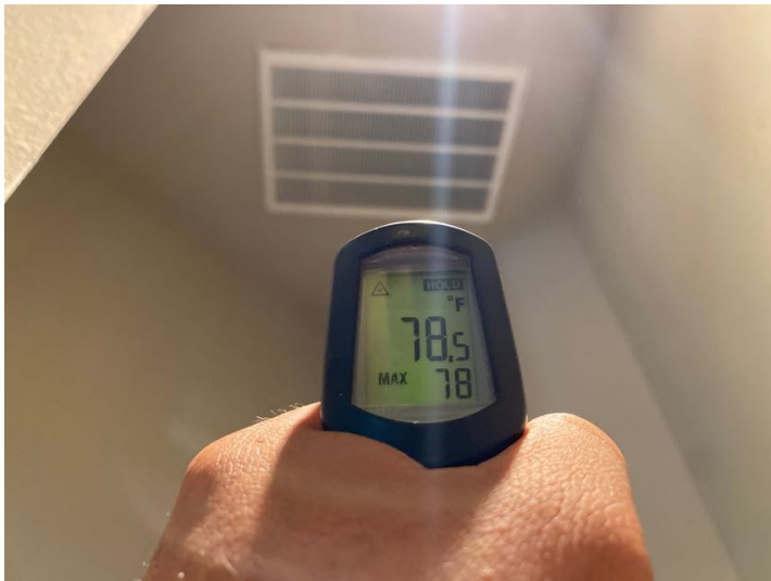
Delta T test at the return vent(upstairs)
