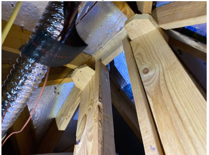
Roof Structures and Attic space
