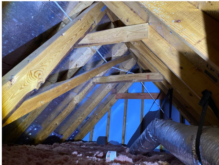
Roof Structures and Attic space
