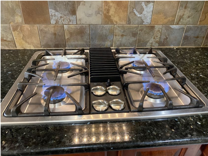
Cooktop:All heating elements operated when tested.
