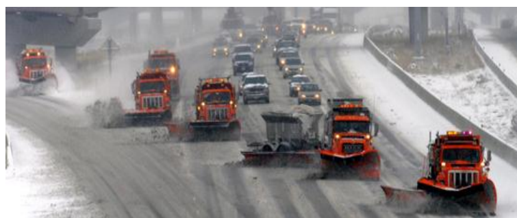
Figure 6 Snow plow working in winter condition for Utah (source: UDOT)
