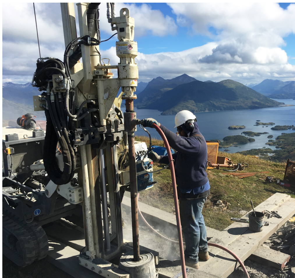
Soni Makihele, Driller, advances air rotary tooling through bedrock on a remote mountain top. The 6712DT was mobilized via helicopter long line.
