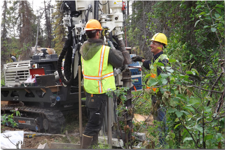
DJ Wardwell, Assistant Operations Manager/Driller, and Scott Bombard, Driller's Helper, both with Discovery Drilling, advance 4.25 in. hollow stem augers to install 2.0 in. groundwater monitoring wells with the 6712DT.
