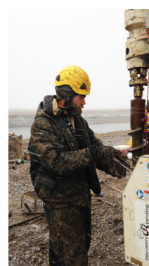
Derek Dell, Driller for Discovery Drilling, advances 3.25-in. hollow stem augers using the GA2500 auger on the 6712DT.
