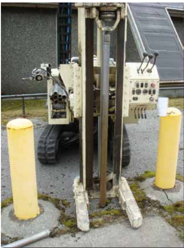
Many of Discovery Drilling's clients specifically request their Geoprobe® rigs because of their small footprint and the ability to access tight spaces.
