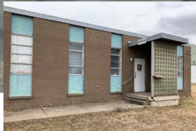
Figure 9 - Current Photo of Office Space
