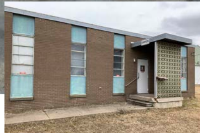
Figure 22 - Current Photo of Office Space
