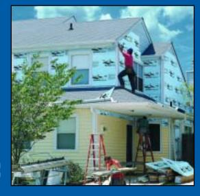
Adding STYROFOAM brand insulation during the residing process is quick and easy.
