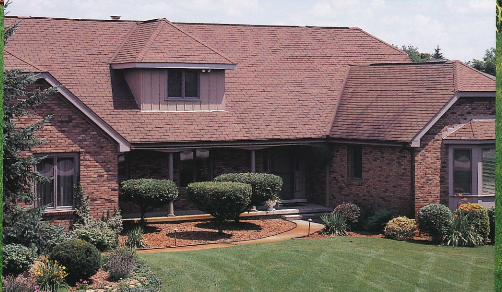
Before Oakridge 40 AR shingles were installed, this beautiful home was covered with a drab, uninteresting roof.
