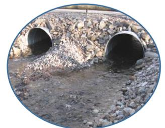
The WLA, through a generous donation from the Alastair and Diana Gillespie Foundation, contributed \$1500 towards the cost to replace two failing 4-foot culverts on private property along Scanlan Creek with twin 5-foot culverts. Installed last summer, the
