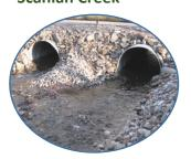
The WLA, through a generous donation from the Alastair and Diana Gillespie Foundation, contributed \$1500 towards the cost to replace two failing 4-foot culverts on private property along Scanlan Creek with twin 5-foot culverts. Installed last summer, the
