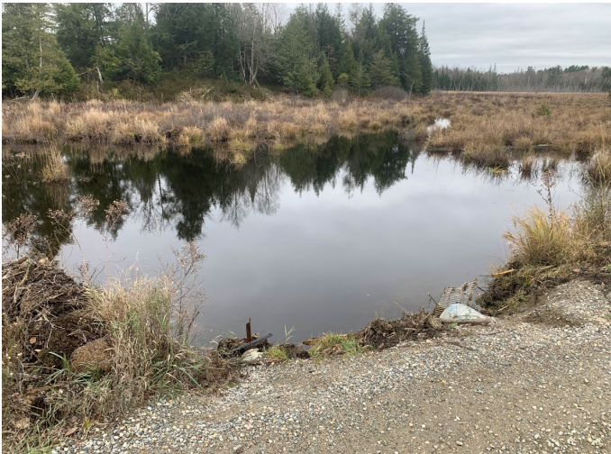
Culverts at Clark Road and south wetland
