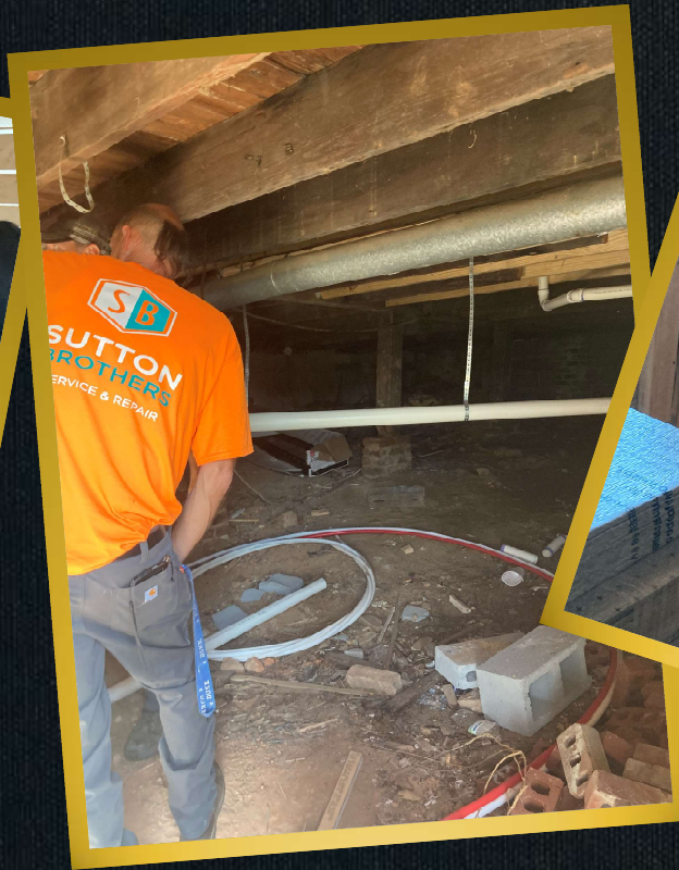
Plumbing under house
