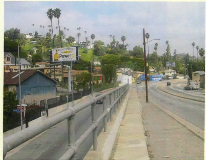
View from Soto Street Bridge Looking North
