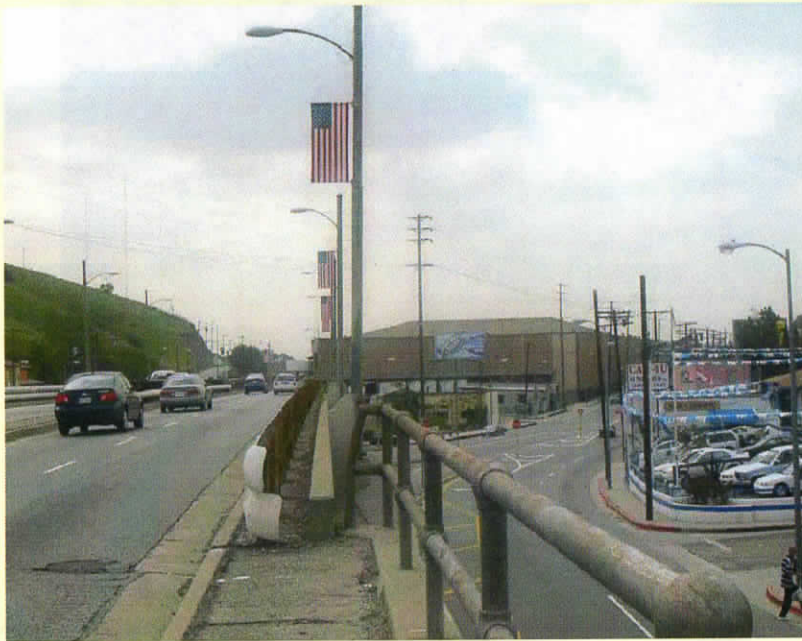
View from Soto Street Bridge Looking South
