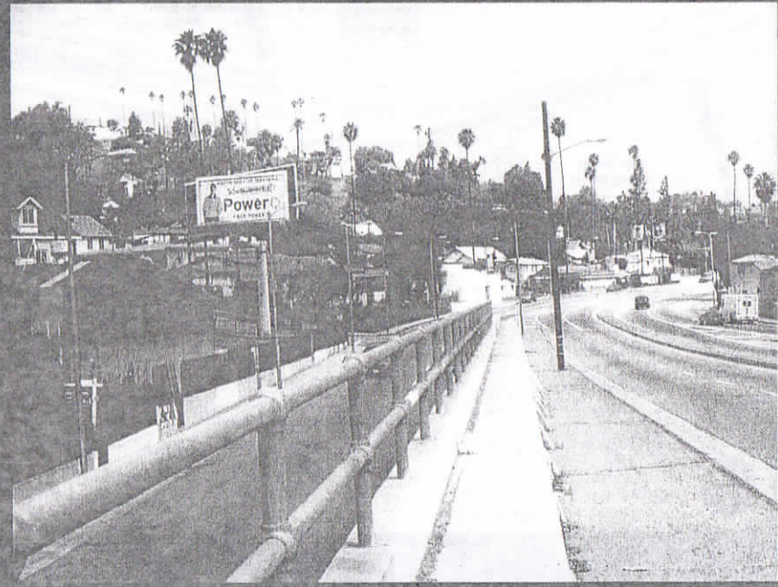
View from Soto Street Bridge Looking North
