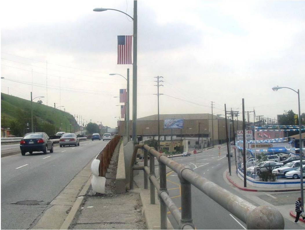
Photo 3: View from Soto Street Bridge Looking South
