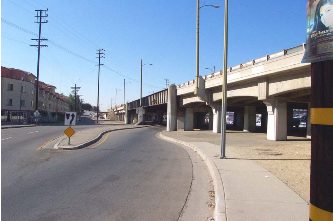
Photo 1: Soto Street Bridge Looking South from Huntington Drive South
