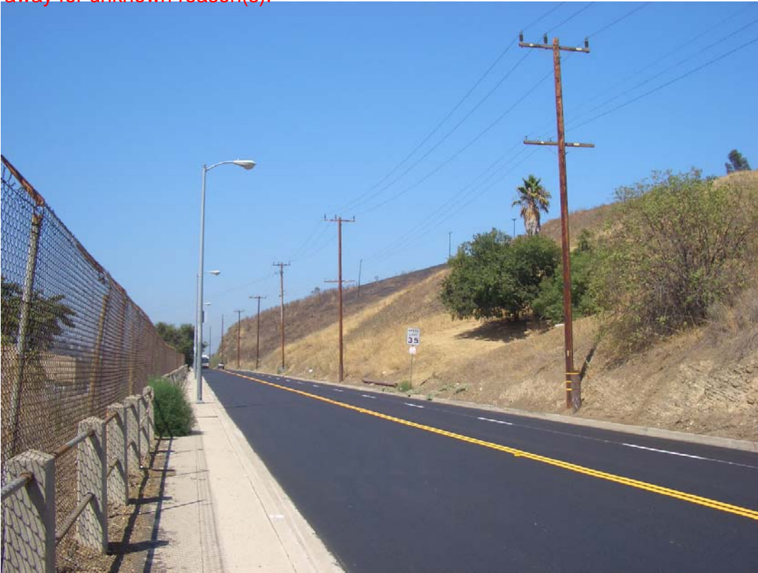
Photo 3: Facing north on Soto Street from a location north of the intersection of Soto and Multnomah Streets, looking from the west side of the roadway. Note the single southbound lane and the two northbound lanes. The hillside east of Soto Street is proposed to be used for roadway widening. Relocation of the overhead electrical wires may be
