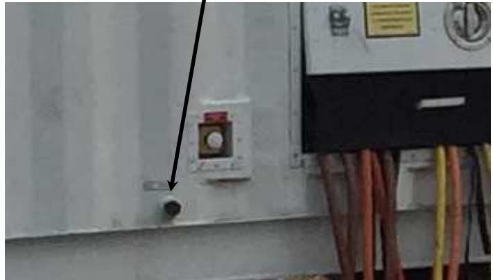
External fuel drain fitting.
