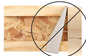
Hanger not plumb
