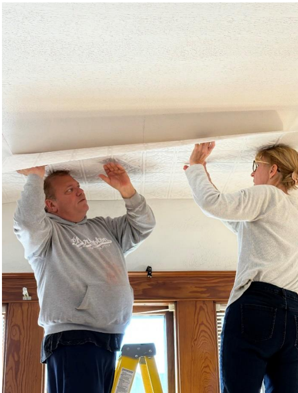
Darren Kauk and Deb Perez install the ceiling.
