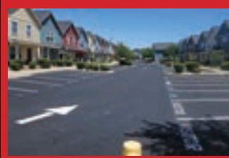
Parking Lot Striping
