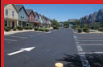
Parking Lot Striping
