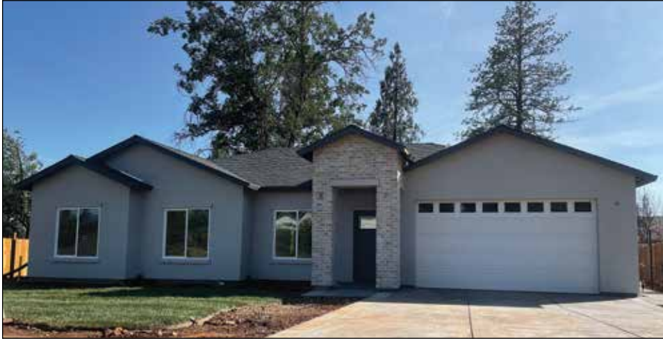
One of Paradise’s many spec homes now under construction all over the ridge.
