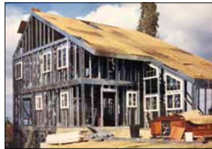
House under construction, California / © Mike Roddy
