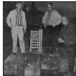
Paradise Post, 1968: scale model of the 1972 sign atop the massive timbers used in the sign’s construction.
