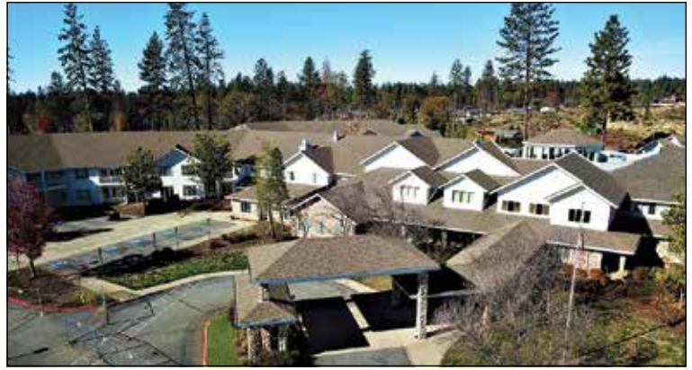
A birdseye view of the Boutique Apts. facing the West Feather River canyon
