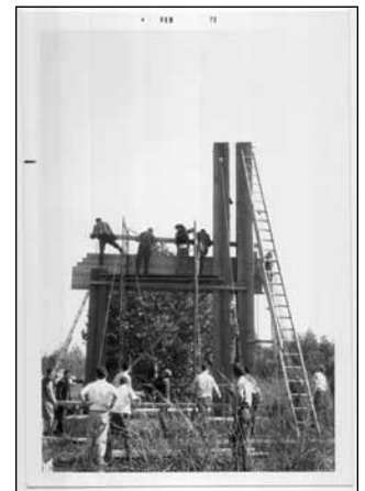
Construction of the original halo sign, February 1972.
