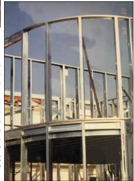
House under construction, California / © Mike Roddy
