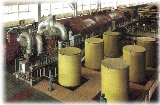
Above: Kingsnorth 500,000kw Turbogenerator
