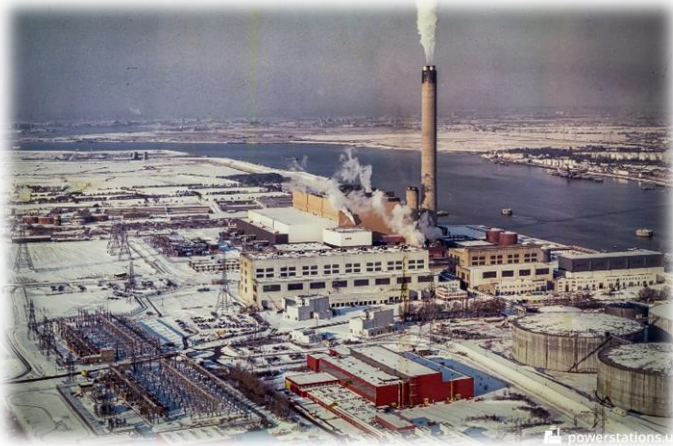
Above: Littlebrook Power D station at full load on a snowy winter's day
