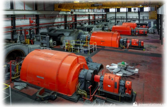
Above: typical emergency gas turbine generator arrangement
