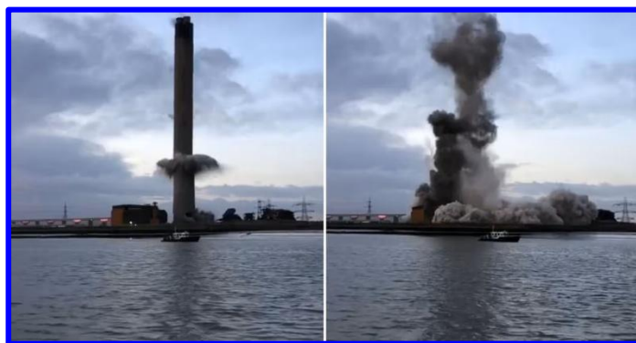
Above: Littlebrook D Power station ends as its chimney is demolished
