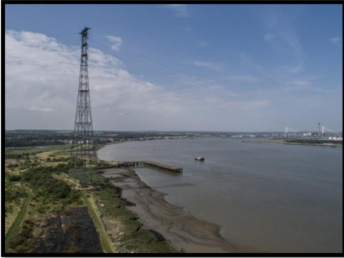
Above: the 400 KV Thames Crossing tower in Kent
