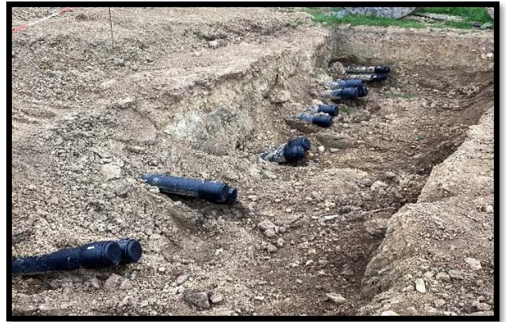
Ducts emerging from the directional drill locations
