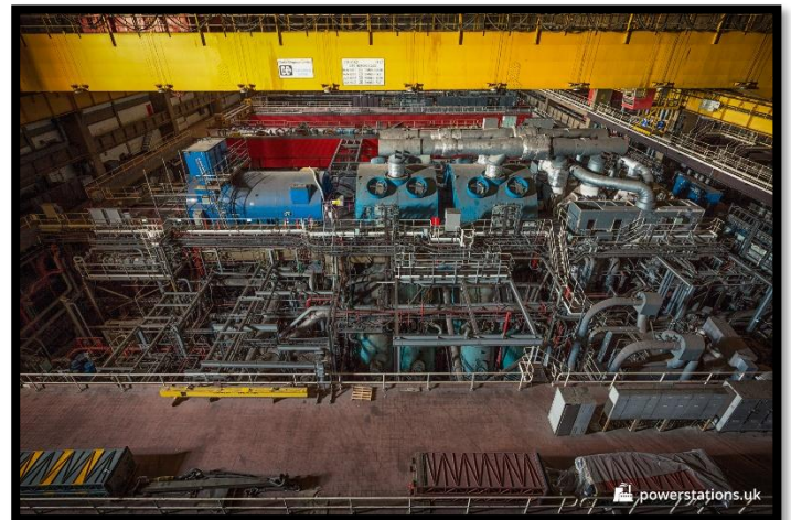
Above: ariel view of Unit 3 being built
