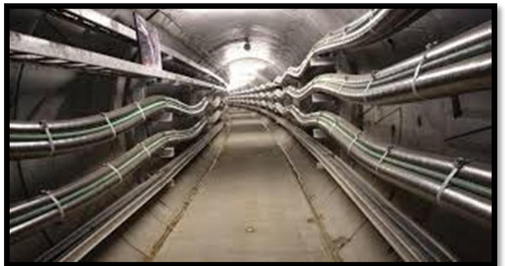
Above: a typical power station cable tunnel
