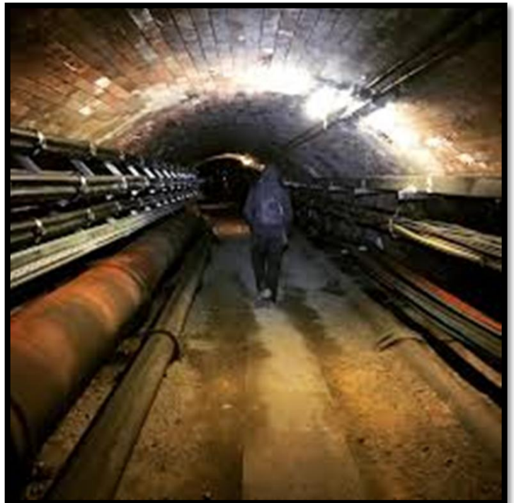
Above: a typical able tunnel under a power station
