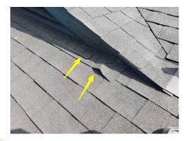
10: Shingles are not installed over the sides of flashing(s).
