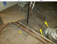
**66:** There is debris and/or insulation in the safety pan that should be cleared out.
