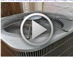
**64:** The outside a/c unit fan electrical wires are exposed above the cover.
