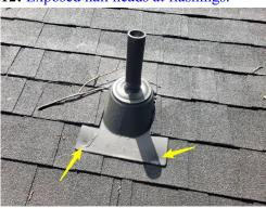
13: There is evidence of previous repairs on sections of the roof.
