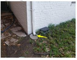
**15:** The gutter at the rear is missing a downspout and an end cap.
