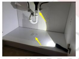
**85:** The main drain and sewer line cleanouts were not found. The type of material for the main drain (and drains under the house) is not known, but could possibly be older cast iron drains - a section of cast iron was observed at one of the bathroom sinks inside the wall.
