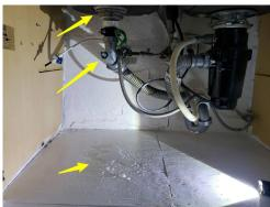
**84:** The hall bathroom sink drain connections also leaked slightly. Sinks are filled water then drained.
