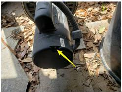
111: The pool light did not work at the time of inspection. The light is also loose at the pool wall.
