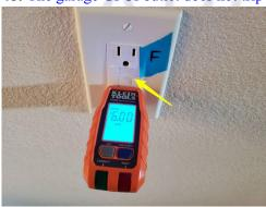
**49:** The exterior outlet/switch near the pool does not work. This outlet/switch is also not watertight (completely loose at the box).
