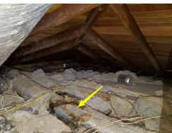
71: There are two abandoned returns (one could have been a supply register) in the living room. It is not known if these are properly sealed/terminated in the attic.
