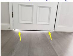
**26:** The doors labeled "A" need minor adjusting/trimming to properly close.
