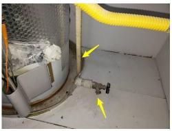
**92:** The water heater T&P valve drain line also does not extend to the exterior of the house (terminates in the safety pan).
