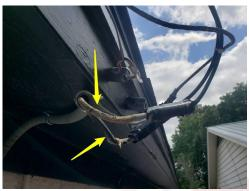
**41:** The service wires do not have adequate clearance from the ground. The wires are very low and are within arms reach (the service head is installed below the roof line).
