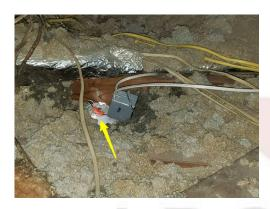
**46:** One of the rear exterior light fixtures is also poorly wired. Wired are exposed, and it seems that connections are covered with a bicycle tire tube.
