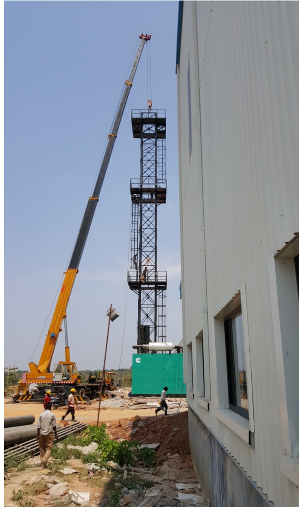
150 feet Chimney structure work, Poonapalli
